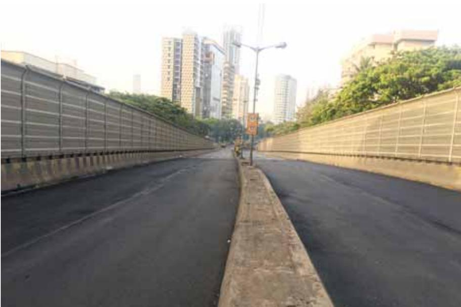
**ABOVE:** This is one of four sections of Mumbai's expressway which has been surfaced with Kraton Polymer's HiMA (highly-modified asphalt)
