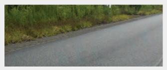
NCAT Section N8 with 140 mm (5½") HiMA rehabilitation after 13 months, 5.3 MM ESALs. Oklahoma sponsored this section through the 2012 test track cycle to monitor deterioration and evaluate preservation strategies. The pavement lasted 16 MM ESALs.
