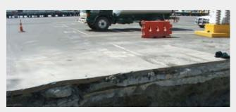
A container loading area in the port of Napier, New Zealand had a severe pavement rutting.
