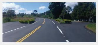
The highway achieved 45 percent thickness reduction after 30.5 cm. (12 in.) of old asphalt pavement were replaced with 16.5 cm. (6.5 in.) of HiMA.
