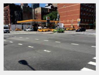
In 2014, First Avenue received the resurfacing. A high performance thin overlay (HPTO) mix with HiMA was used. After three years, the road is still in a great condition, making First Avenue safer, quieter and more attractive.
