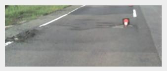
The NCAT Section N8 conventional rehabilitation after 10 months, 4 MM ESALs. The 250 mm (10") pavement was paved in August 2006, and a 125 mm (5") rehabilitation was done in August 2009. The first crack appeared at 2.7 MM ESALs.
