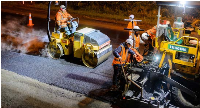
Higgins places HiMA lift on Kapiti Expressway, S.H. 1 at Lindale Village
