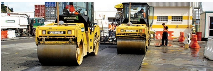
Surface wearing course placed following HiMA base layer
