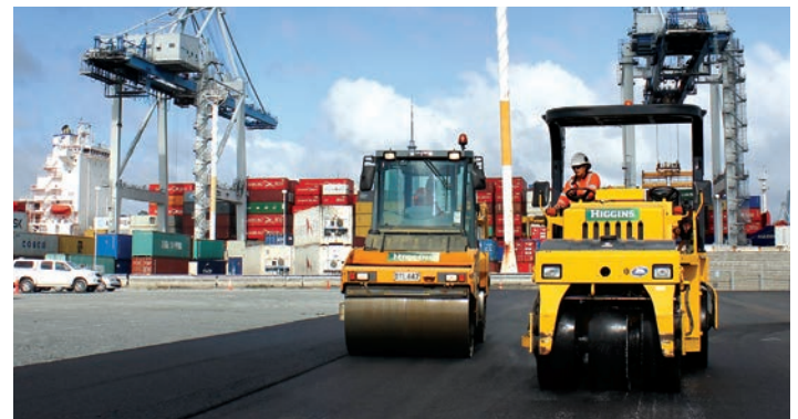
Higgins compacts section incorporating HiMA at Port of Auckland
